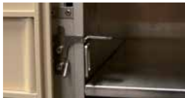
Easy release handle to open master gate
