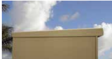
Sloped top for moisture runoff
